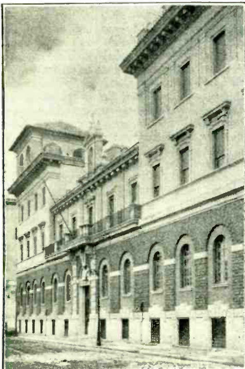
The new broadcasting building in Rome. It includes eight studios, one of which is used exclusively for television.
